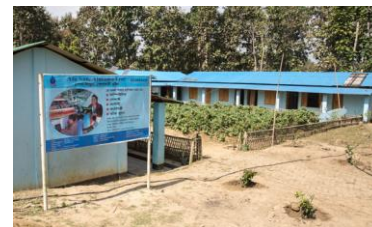
The vocational school in Thanchi It comprises three school buildings, a residential home and a workshop for the weaving course.
